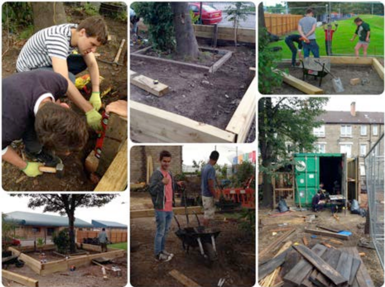
Fig. 3. Construction of the sandpit at Baltic Street Adventure Play
