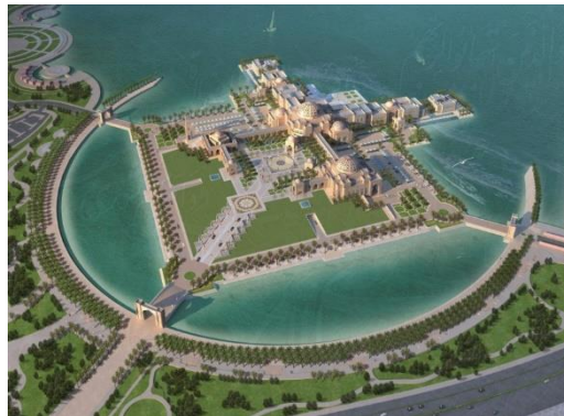
Figure 4, The National Assembly project, Kingdom of Bahrain
