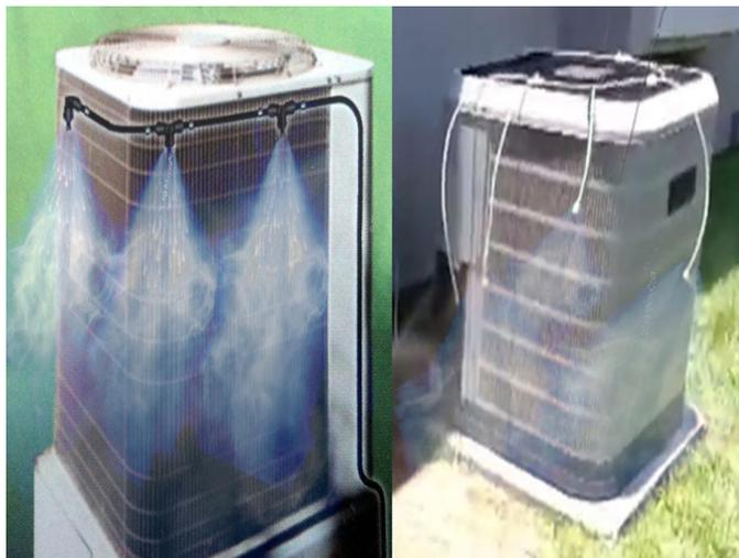
This system comprises pump, mist nozzles, piping arrangement and temperature control. As the temperature reaches the set point the thermostat will turn on the pump.
