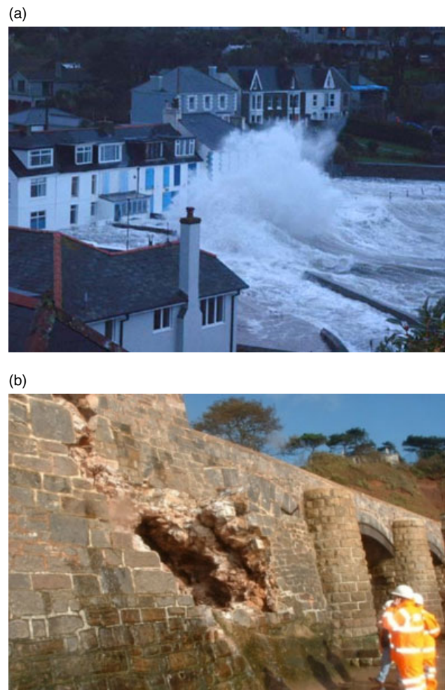
Figure 1. (a) Storm-induced wave overtopping at Portmellon, Cornwall (Photograph by Marie Preece). (b) Storm damage to the sea wall protecting the mainline railway between Dawlish and Teignmouth. © Network Rail. This figure is available in colour online at wileyonlinelibrary.com/journal/gj
