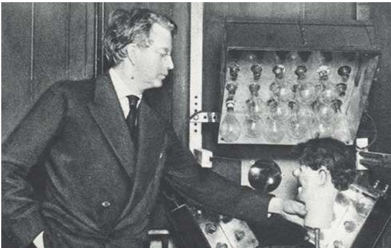
Figure 2: Baird with his transmitter, believed to be that used for the first demonstration of television in 1926.[14] One of the 30 lenses can be seen to the left of the dummy's head mounted in a plywood, 1.5m diameter scanning disk.[4, p.55]
