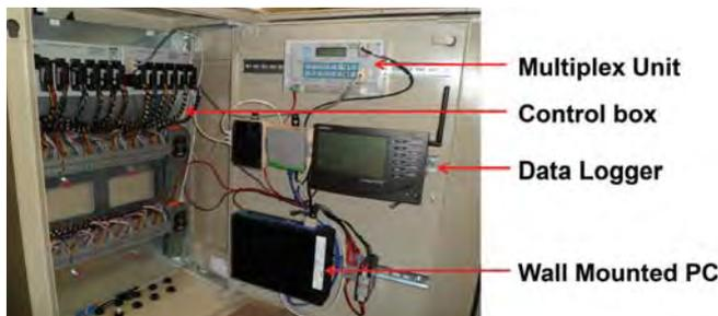
Figure 11: Instrumentation.
