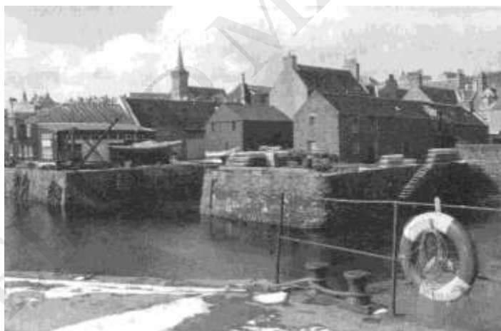
b) The original buildings in 1930
