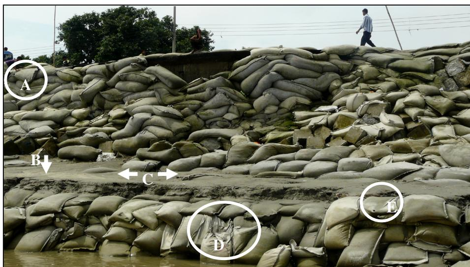
A: Plug, B: Slump, C: Missing top, D: Sliding and E: Physically damaged
