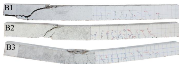
Figure 5. Crack Patterns after Failure
