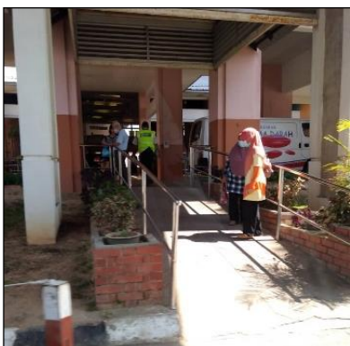
Figure 9. Handrail at Hospital A
