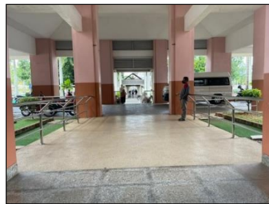
Figure 8. Ramp at Hospital B
