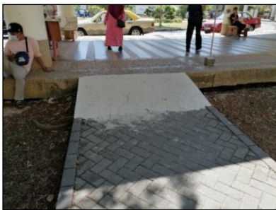
Figure 7. Ramp at Hospital A
