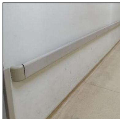
Figure 10. Handrail at The Entrance of Hospital B
