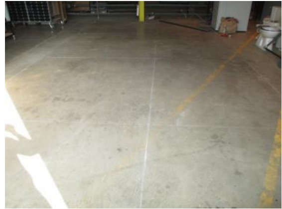
Figure 7. Drainage Lab slab studied in this work.
