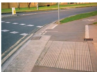
Figure A5. Tactile paving
