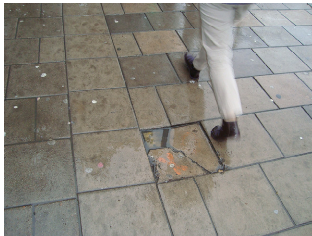
Figure 6. Cracked paving flag and wet conditions
