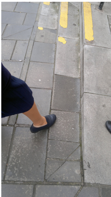
Figure 5. Changes in levels – tapered steps require greater concentration and are a source of stress
