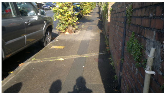
Figure 2. Changes in levels – drain across pavement
