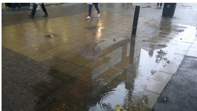
Figure 13. Accumulation of water during wet weather conditions may increase slip risk
