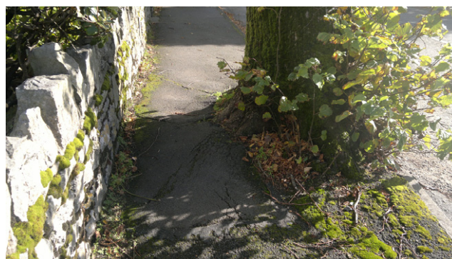
Figure 7. Bitumen surface made uneven by tree roots
