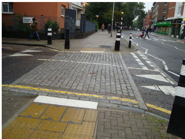
Figure 9. Tactile paving and setts are uncomfortable and can lead to imbalance
