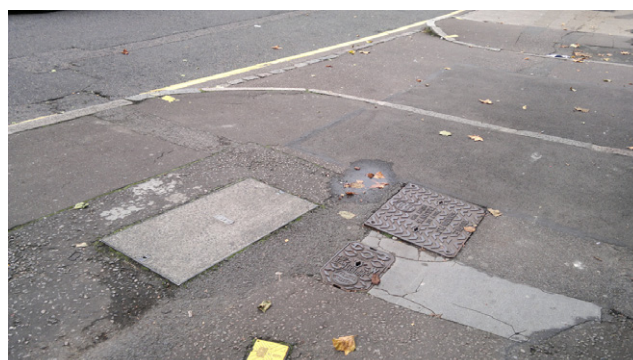
Figure 3. Changes in levels due to manhole covers
